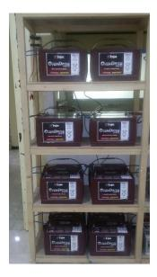
Due to the rapidly increasing power disruptions, Saba Islamic Bank has an emergency generator. The generator takes few seconds to start. To prevent the servers from being shut down while the generator is starting, a power bank was installed. The Power Bank was connected to a 10 KVA inverter used as an emergency backup system for the bank's servers.
